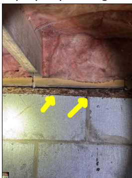
Rust/corrosion along the metal plate against the sill. This is an indication that the crawl space has an active or intermittent water source. An active or intermittent water source can cause mold growth and property damage, such as wood rot, rust, and corrosion.
