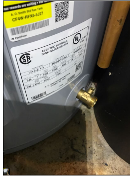
Water heater data plate.
