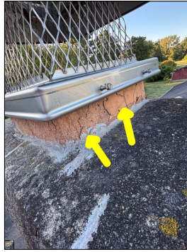
Cracks along the clay tile. Cracks along the clay tiles are a potential safety hazard. Cracked tiles can cause the chimney to not draft properly, thus potentially causing carbon monoxide to enter the house or potentially cause a fire.
