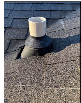
The plumbing vent is unconventionally short. This is considered abnormal and a defect. A short plumbing vent can get covered during heavy snowfall, thus obstructing the vent, which could result in drainage problems with the plumbing system.
