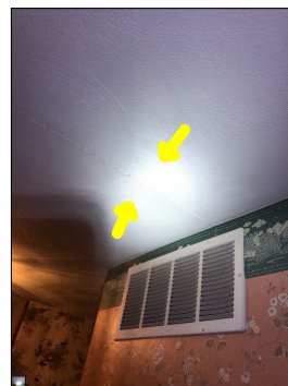
Cracks along the ceiling.
