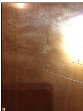
Damage/dents along the door.
