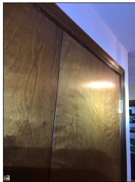
The doors rubs each other during operation.
