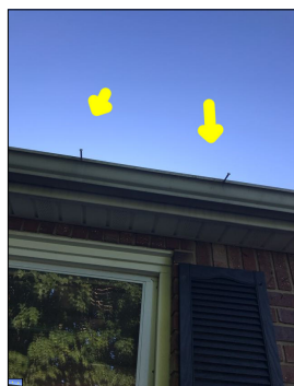
Loose gutter spikes.
