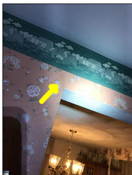
Cracks along the walls.
