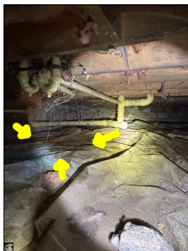
Moisture and dampness observed underneath the plumbing lines. The water source could potentially be from a leaking pipe or from ground water. Recommend general contractor further evaluate and make necessary repairs.
