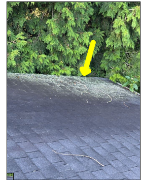
Biological growth along the roof. This is considered a defect. Biological growth has the potential to hold water. Shingles are not designed to hold water, shingles are designed to shed water.
