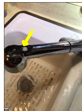
The button pad is deteriorated.
