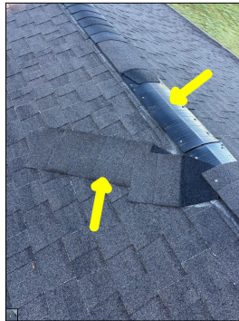
Loose/detached roof shingles. This is considered a defect and a potential leak point.
