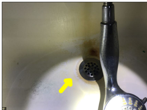
Cracks along the bathtub.
