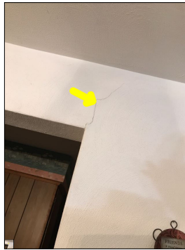
Cracks along the walls.
