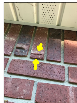
Cracks along the siding.
