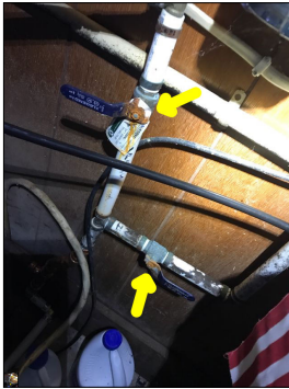
Corrosion and rust along the valves.
