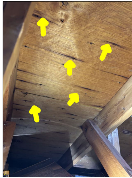
Black discoloration around the roofing nails and black discoloration around previous holes from prior roof shingles. The black discoloration is a potential mold like substance. This is caused by an active or intermittent water source. In most cases, the discoloration is caused by inadequate attic ventilation. An active or intermittent water source can cause mold growth and property damage.
