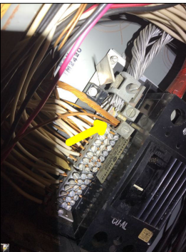
Different gauge wires within the same terminal. This is a potential safety hazard. The different size wires within the terminal can create a poor connection, thus causing spark, arcing and/or fire.
