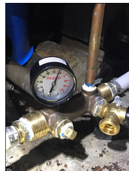
The well pressure was approximately 58 PSI during the inspection.
