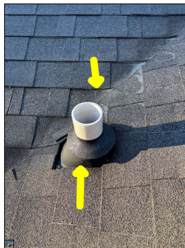
Unconventional flashing/roof penetration along the valley . This is considered abnormal and a potential leak point. The roof penetration is too close to the valley for modern day roofing standards. There should be at least 18 inches from side to side from the middle of the valley. Due to the unconventional location of the roof penetration, this area is a potential leak point.
