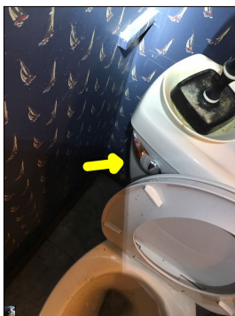
The handle is unconventionally loose.
