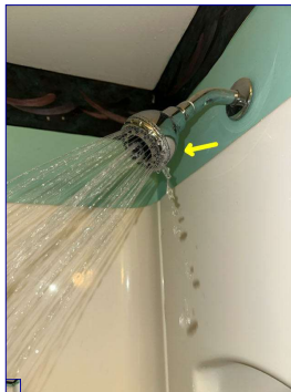
The showerhead is leaking. Recommend a licensed plumber replace as needed.
