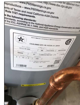
Water heater data plate.
