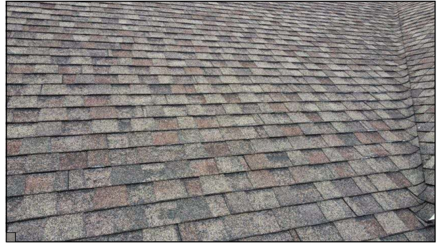
Granule loss along the roof shingles
