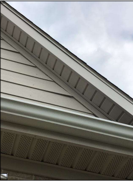
Warped panels.
