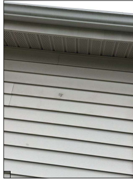
Discoloration along the siding.
