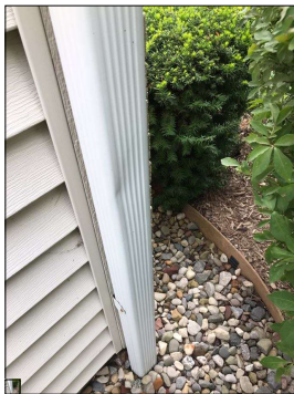
Dents/damage along the gutter system.
