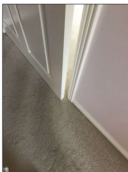
The door drags the floor during operation.
