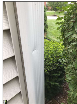
Dents/damage along the gutter system.
