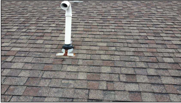
Rust and corrosion along the flashing. Rust and corrosion can create holes in the flashing, thus creating potential leak points.
