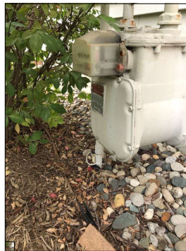
Main fuel shut off valve.
