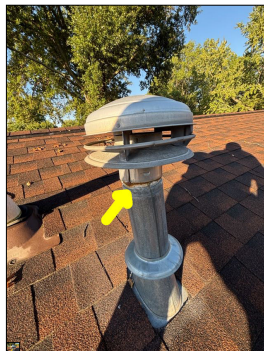
Rust and corrosion along the flue. Rust and corrosion can create holes along the flue, thus creating potential leak points.
