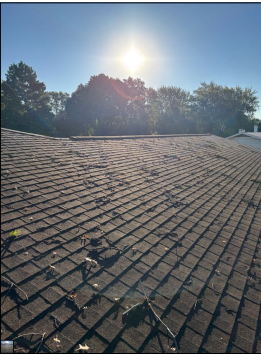
General photo of the roof.
