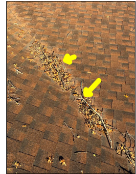
Debris along the roof. Excessive debris along the roof can restrict the ability of the roof to shed water, thus creating potential leak points.
