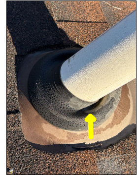
The rubber flashing is concave. This is considered a defect. The concave flashing will act as a trap for water and hold water and snow, thus creating a potential leak point. Flashing is not designed to hold water, flashing is designed to shed water.
