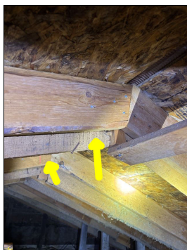
Sistered trusses observed in the attic. This is an indication of previous structural repairs.
