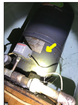
Mold like substance along the pressure tank. An active or intermittent water source can cause mold growth and property damage.
