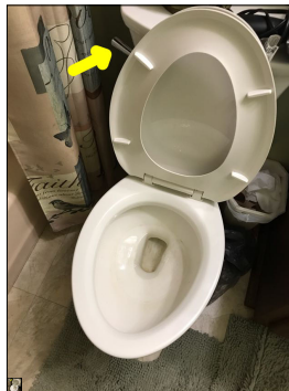
The lever has to be held down for a few seconds for the toilet to flush. This is considered abnormal and a defect. A toilet should properly flush by simply pressing down on the lever and then releasing from the lever.
