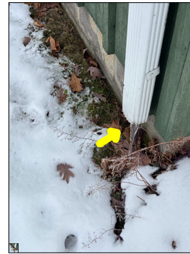
Missing downspout elbows.
