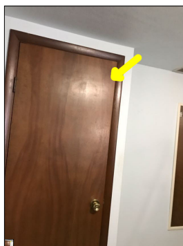
The door rubs the frame during operation.
