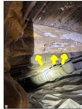
Wood rot damage observed. Wood rot is caused by a wood-decaying fungi.
