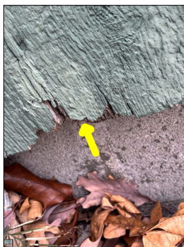
Deterioration along the siding.
