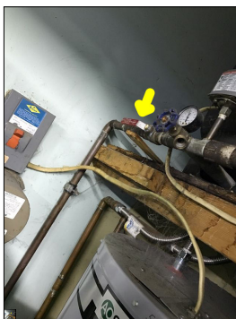
Apparent main water shut-off valve.
