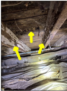
Mold like substance along the subfloor and floor joist. An active or intermittent water source can cause mold growth and property damage.
