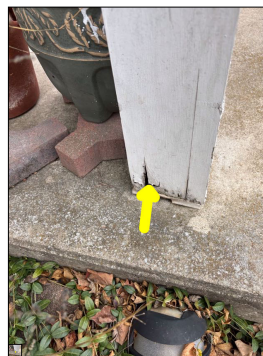
Wood rot damage along the columns.
