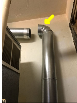
Detached ductwork.
