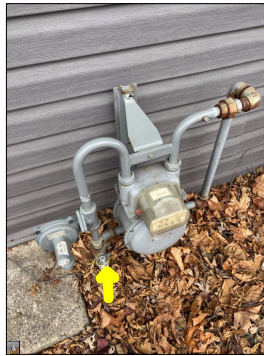
Main fuel shut off valve.
