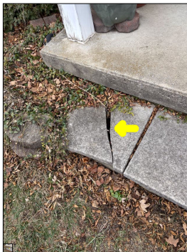
Cracks and deterioration along the service walks.
