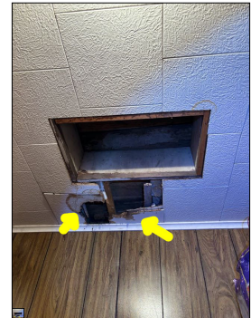
Discoloration and signs of previous water damage. An active or intermittent water source can cause mold growth or property damage.
