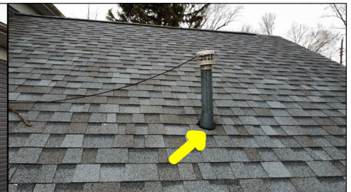
Unconventional application of sealant along the roof. This is considered abnormal and amateur craftsmanship. Amateur craftsmanship is prone to failure and leakage.
