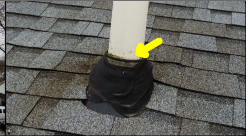
Unconventional rubber coupler observed along the vent pipe and unconventional flashing. This is considered abnormal and a potential leak point.
