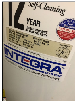
Water heater data plate.
