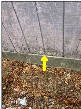
Deterioration along the siding.
