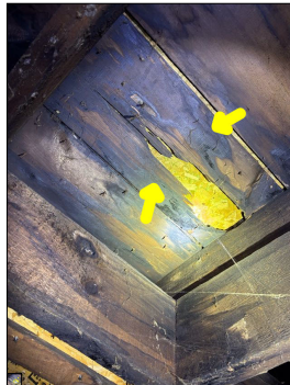
Discoloration and deterioration along the sheathing. An active or intermittent water source can cause discoloration, mold growth and property damage.
