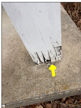
Wood rot damage along the columns.
