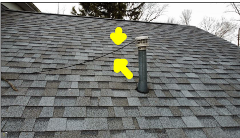
Unconventional cord routed along the flue. This is abnormal and a potential fire hazard.
