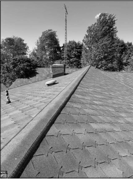
General photo of the roof.
