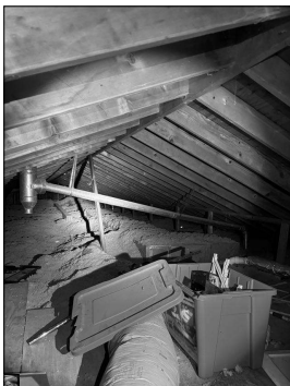
General photo of the attic.
