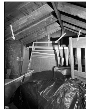
Debris and clutter within the attic. Visibility and accessibility were limited.
