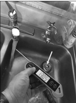
Temperature reading of the hot water during the time of the inspection. The approximate temperature of the hot water was 130 degrees Fahrenheit.
