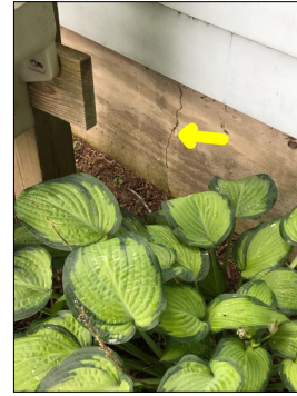
Crack along the foundation. Cracks are considered a defect.
