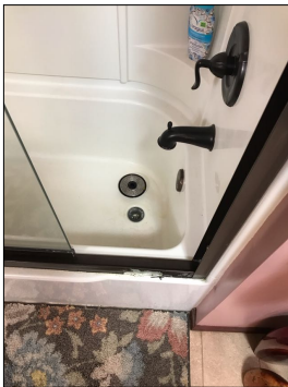
Missing drain stopper.
