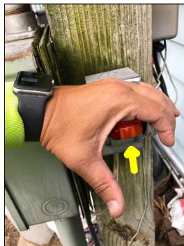
Reverse polarity receptacle.
