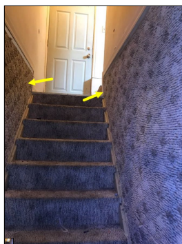
Missing handrail.
