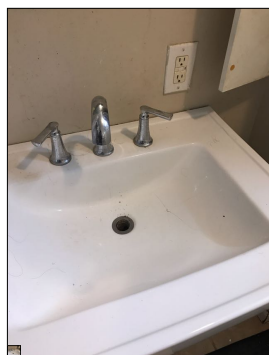
The faucet is inoperable.
