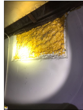
Unconventional application of foam spray along the windows.
