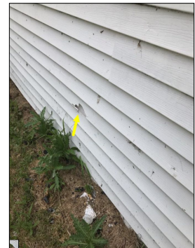
Damaged siding.
