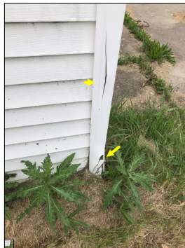
Damaged siding.
