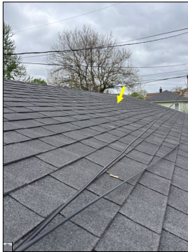
Unconventional waves/sags along the roof. This is considered abnormal and a defect.
