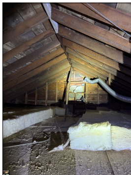
General photo of the attic.
