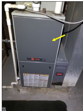
The furnace is inoperable. The burners would never ignite. Only the blower would turn on.
