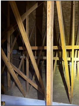
General photo of the attic.
