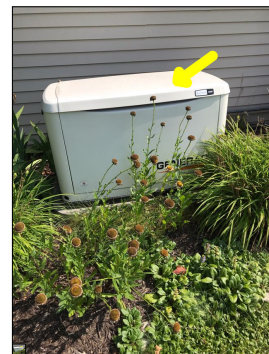
Generator observed. Inspecting generators is beyond the scope of a general home inspection. Generator should have, at minimum, an annual inspection by a licensed electrician and should be operated bi-annually to ensure they are in good working condition. Recommend checking with the seller to see if they have any documents that show annual preventative maintenance has been performed on the generator.
