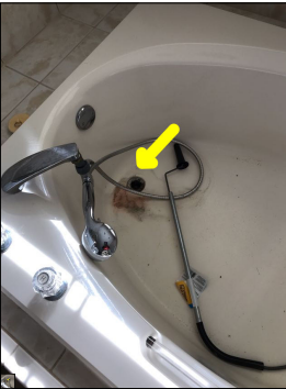
Missing drain stopper.
