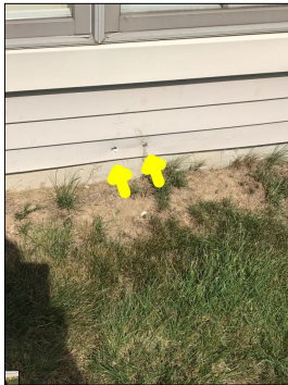
Damaged siding.
