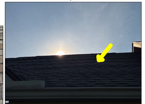
Unconventional waves/sags along the roof. This is considered abnormal and a defect.
