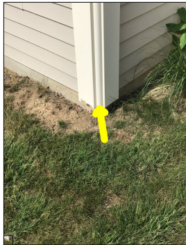
Damaged siding.
