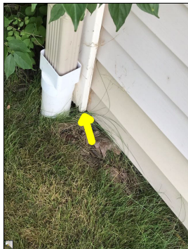
Damaged siding.
