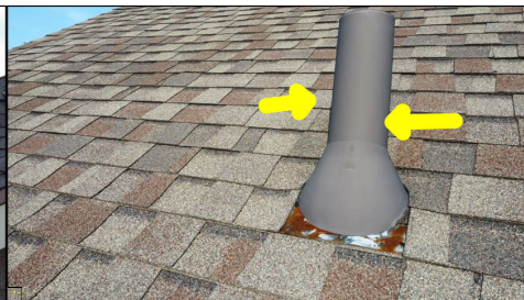
A vent boot repair sleeve (Perma-Boot or similar) has been installed over the plumbing vent. This type of repair is intended to cover a deteriorated rubber vent boot without replacing the existing flashing assembly.
