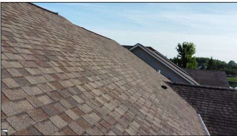
General photo of the roof.
