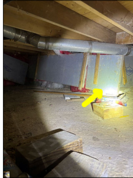
Displaced insulation.
