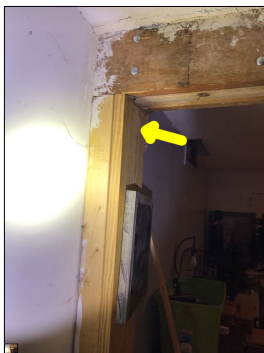
Structural repairs observed.
