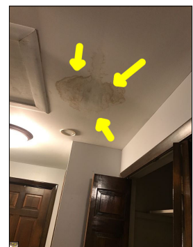
Discoloration along the ceiling and signs of previous water damage. An active or intermittent water source can cause mold growth and property damage.
