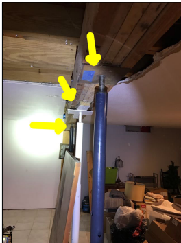
Unconventional alterations and column supports. This is considered amateur craftsmanship. Amateur craftsmanship is prone to failure.
