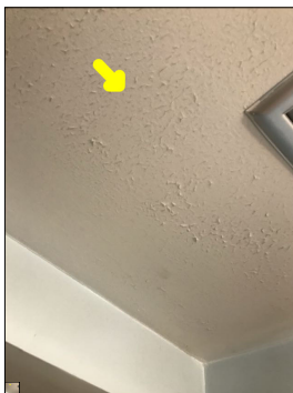
Flaking and peeling along the ceiling.
