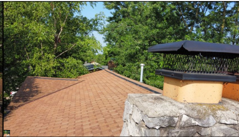
General photo of the roof.
