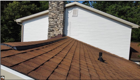
General photo of the roof.
