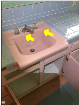
The sink is inoperable.
