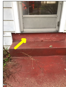
The riser/step is unconventionally high. This is a potential trip hazard. The recommended maximum height for a riser/step is 7 inches.
