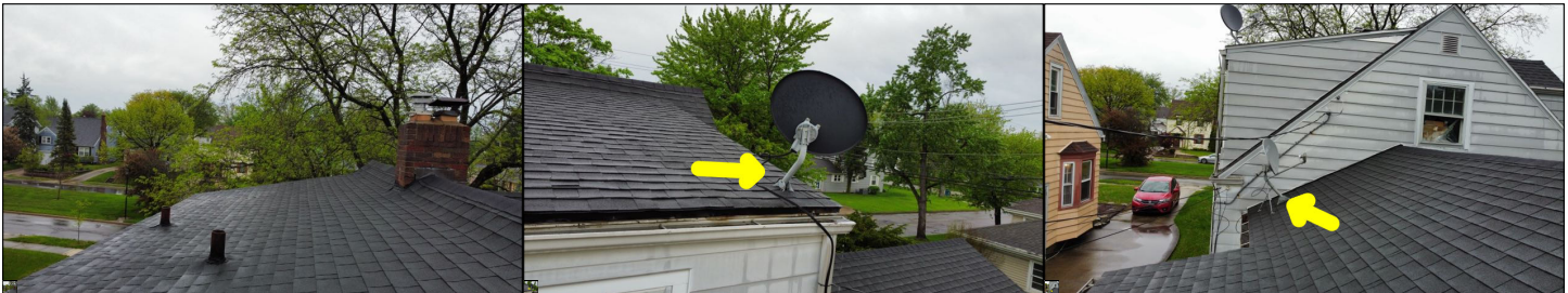
General photo of the roof.
