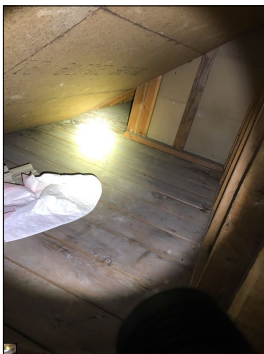
General photo of the attic.
