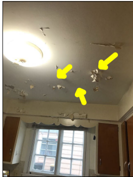
Flaking and peeling along the ceiling.
