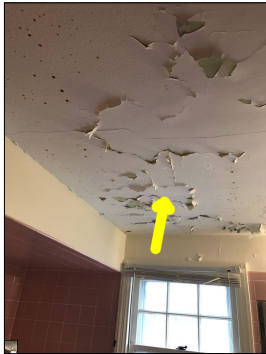
Flaking and peeling along the ceiling.
