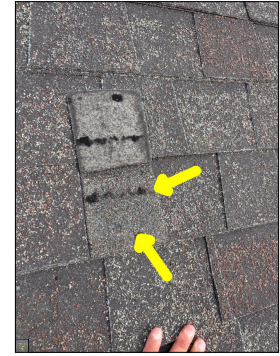
Loose/detached roof shingles. This is considered a defect and a potential leak point.
