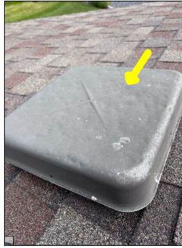
Dents along the roof vents. This is an indication of previous hail damage.
