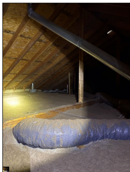
General photo of the attic.
