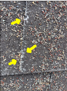
Exposed fiberglass mat along the shingles. This is a sign of deterioration along the roof.
