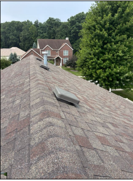
General photo of the roof.
