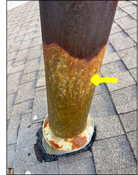
Rust and corrosion along the flue. Rust and corrosion can create holes along the flue, thus creating potential leak points.
