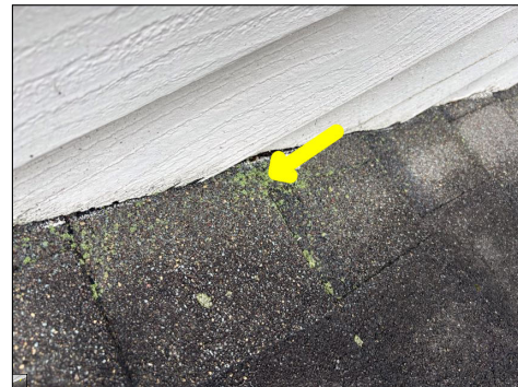
Biological growth along the roof. This is considered a defect. Biological growth has the potential to hold water. Shingles are not designed to hold water, shingles are designed to shed water.
