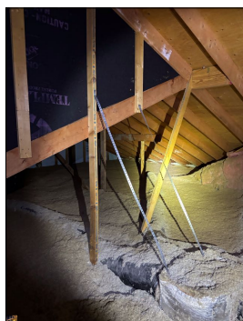
General photo of the attic.
