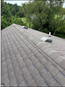
General photo of the roof.
