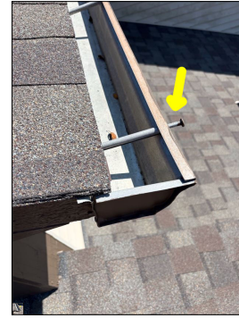
Loose gutter spikes.
