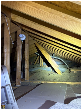
General photo of the attic.
