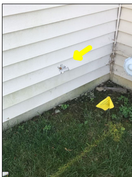
Damaged siding.
