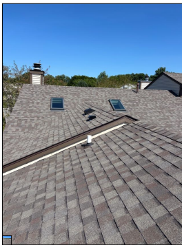
General photo of the roof.
