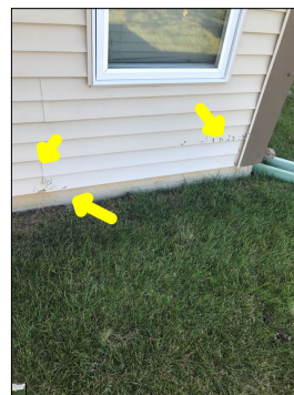
Damaged siding.
