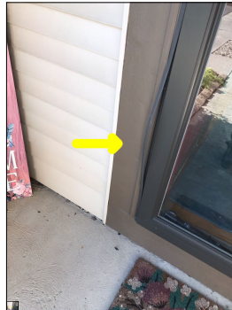
Displaced weatherstrip.
