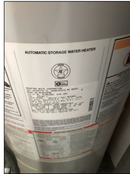
Water heater data plate.
