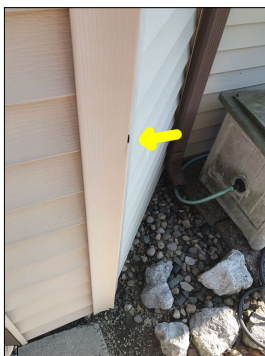
Damaged siding.
