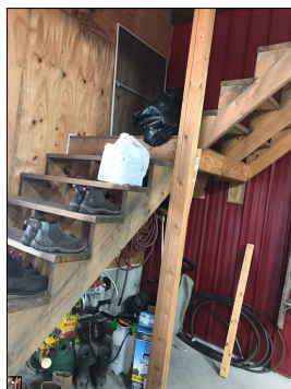
Missing handrail.
