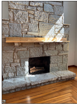
General photo of the fireplace.
