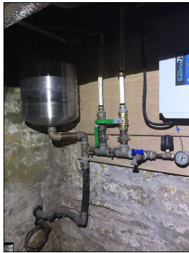
Apparent pressure tank.
