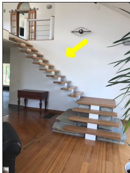
Missing handrail.
