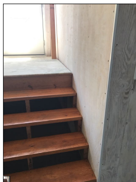
Missing handrail.
