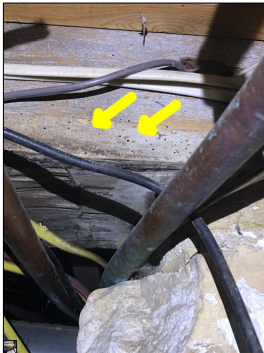
Exit holes observed. Exit holes are an indication of an infestation of powderpost beetles. Powderpost beetles are a wood destroying insect and can cause structural damage and property damage.
