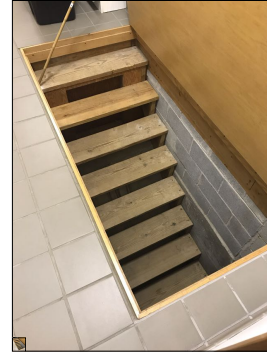
Missing handrail.
