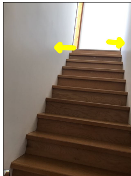
Missing handrail.
