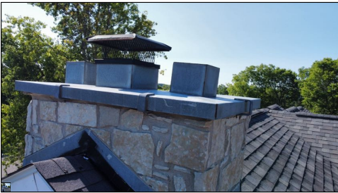
General photo of the chimney.
