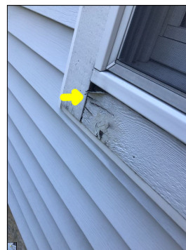
Wood rot damage.
