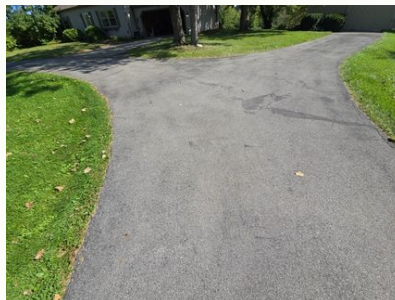
Main asphalt driveway
