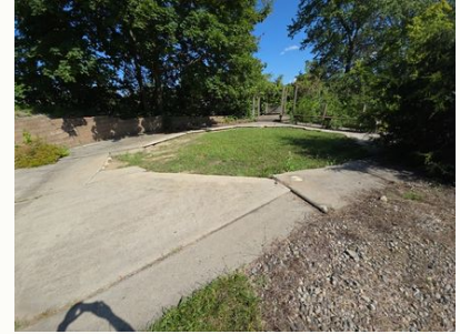
Rear walkway and Patio
