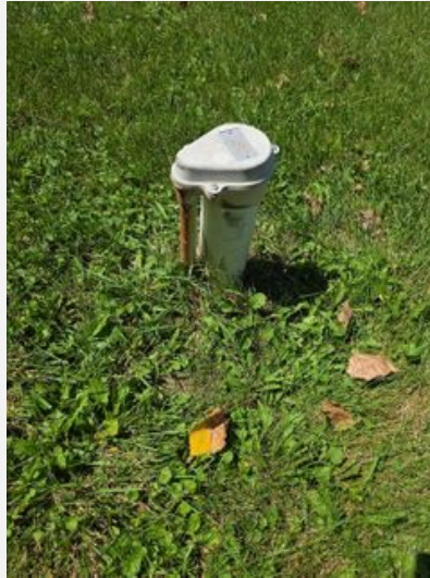
Well cap/head located in the front yard northwest corner
