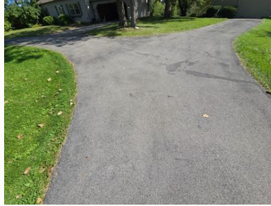
Main asphalt driveway
