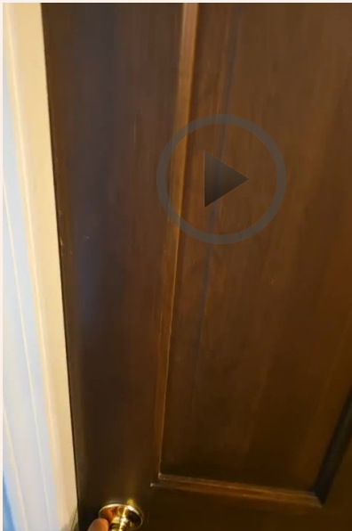
(This video is only viewable online.) Main floor hallway closet closest to the living room is missing door jamb stops
