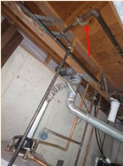
Gas supply shut off to the water heater
