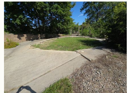
Rear walkway and Patio
